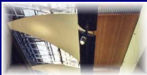
weight sandwich ceiling element of Carbon/phenol > 18 m 2 , total weight 175 kg, including support frame. Total structure is self supporting and carry two persons
